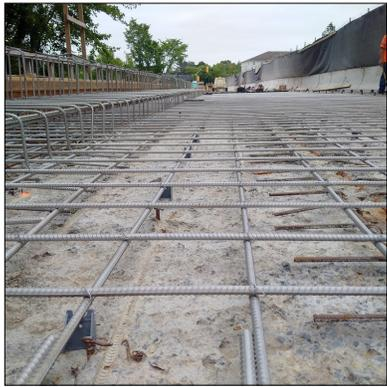
The \$4.8 million dollar rehabilitation of the Nashwaak River Bridge No.1 is included in the New Brunswick government's \$409.5 million dollar investment in roads and infrastructure. Rehabilitation of the bridge was required due to minor vertical cracking in bridge piers and extensive concrete deterioration on the top mat of the bridge deck.
