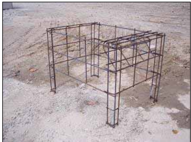
Pre-welded rebar cage.
