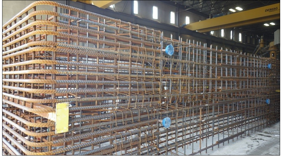
Rebar cages from StelCrete, two cages per delivery, one stacked upon the other
