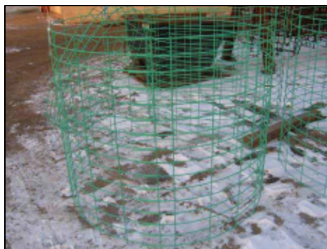
Epoxy-coated cage for maintenance hole component
