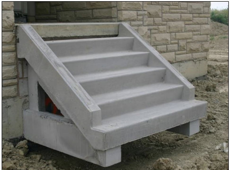
Brick step stair comprised of two side brackets and one riser step assembly
