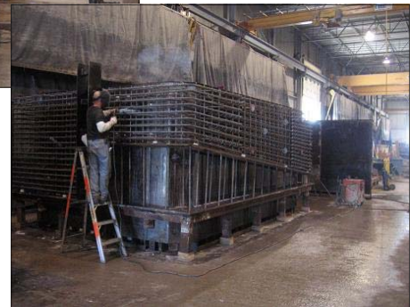
Additional cast-in hardware is connected to the pre-assembled cages.
