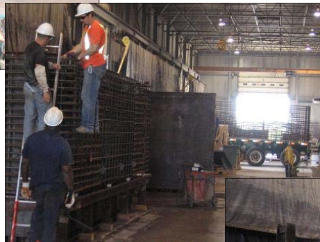
Plant technicians check cover dimensions.
