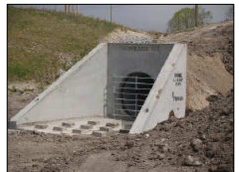
Installed Hanson Quick Headwall.
