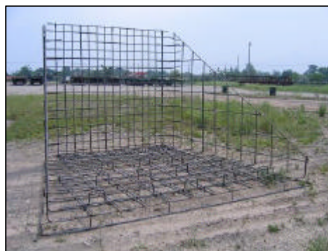
Welded wire assembly for headwall.
