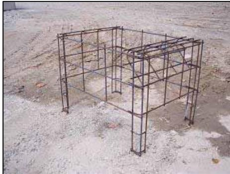
Pre-welded rebar cage.
