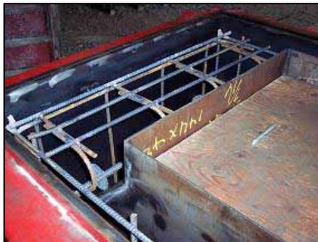
Pre-welded cage placed in transformer formwork.
