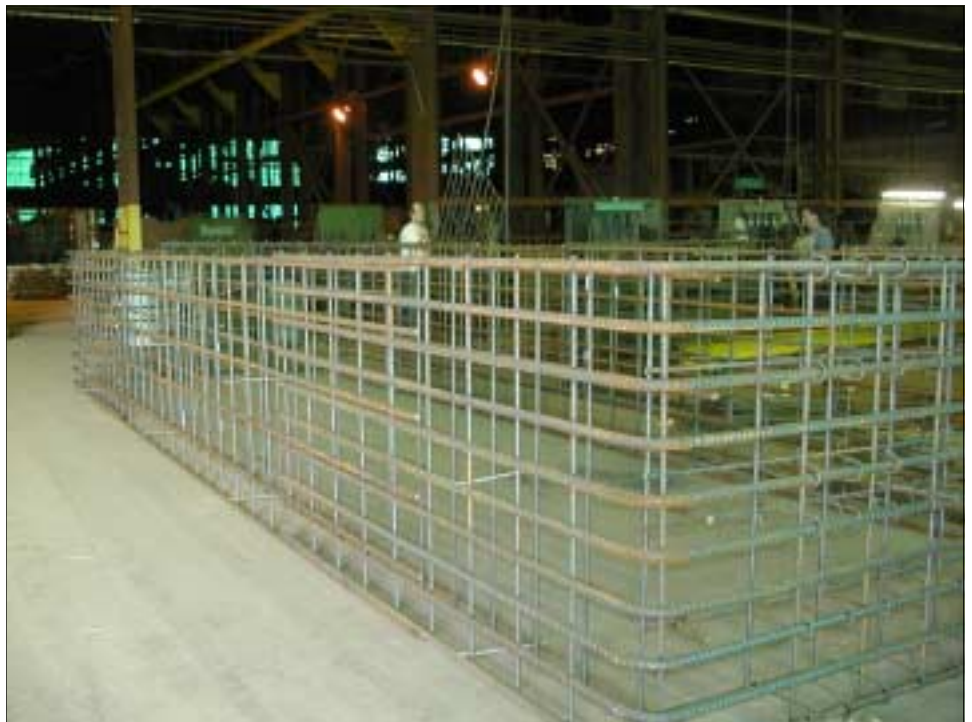
Pre-welded reinforcing assembly with stainless steel stirrups — ready to receive concrete.
