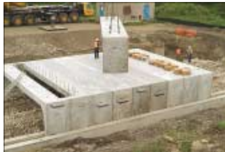
Reinforcement assemblies designed for a light portal in the structure.
