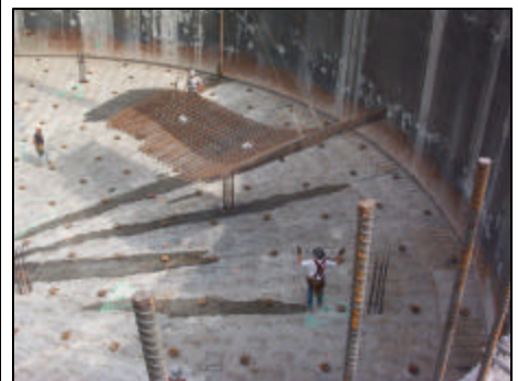
Segment lowered into position
