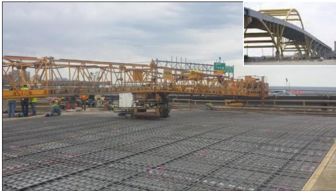
Contractor prepares for bridge deck pour over the #HoanBridge. https://twitter.com/WIHoanBridge
