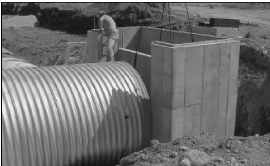
Installing detention facility controlled outlet structure
