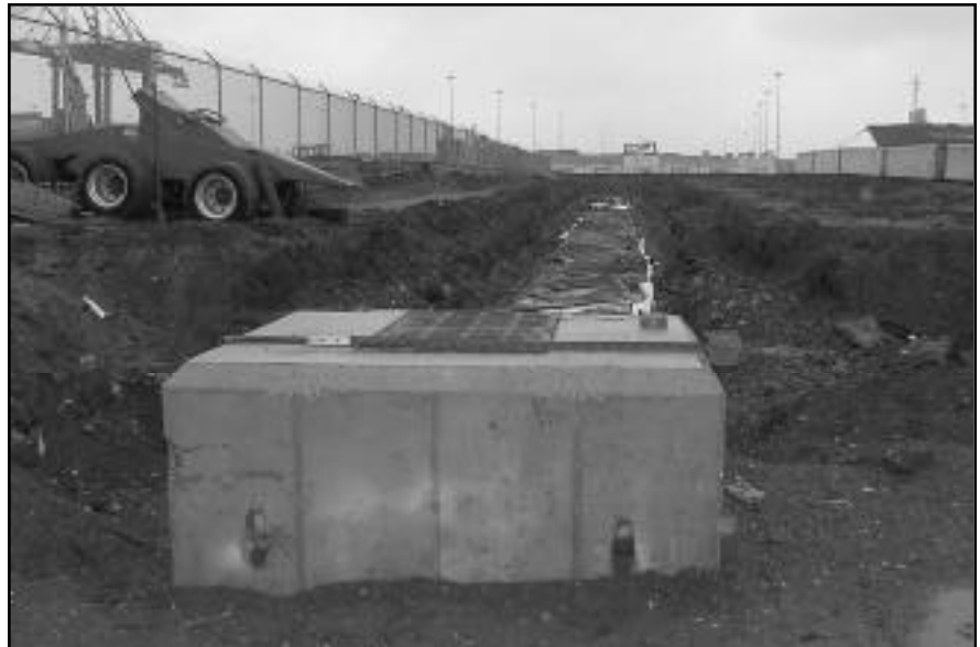
Curing footing for trench runs up to catch basin
