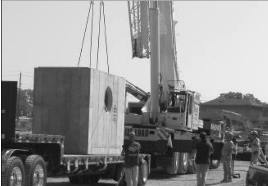
Unloading storm water controlled outlet structure
