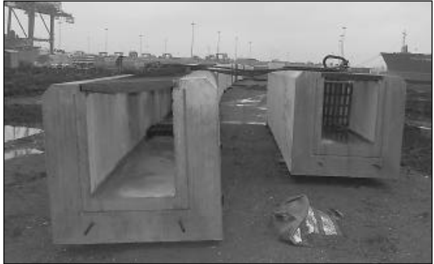
Precast storm water trench units ready for installation
