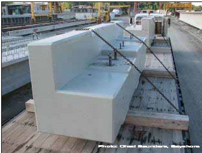
Precast abutments shipped from Bayshore facility to Tangier Island.
