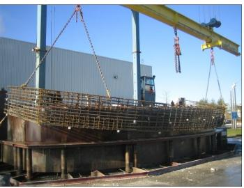
Placement of rebar cage in mold with a span of 10.98m and vertical rise of 3.96m.
