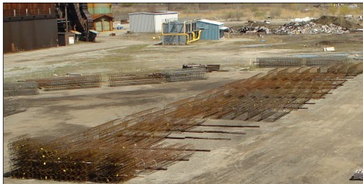
Pre-assembled cages for caissons stockpiled for timely delivery
