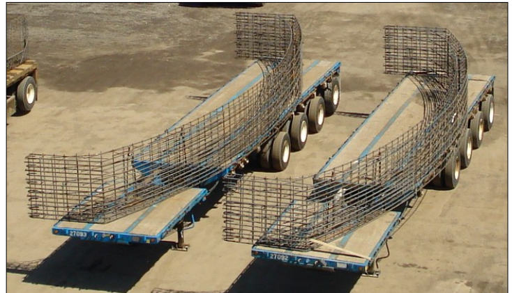
Pre-assembled rebar reinforcement for SUPER/SPAN precast mould
