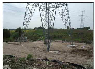
Pre-assembled cages used for poured-in-place construction of tower caisson bases
